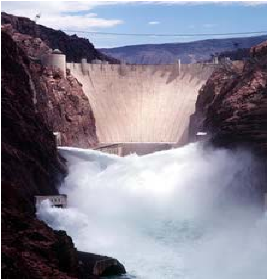
Hoover Dam, United States One of America's "Seven Modern Civil Engineering Wonders"
